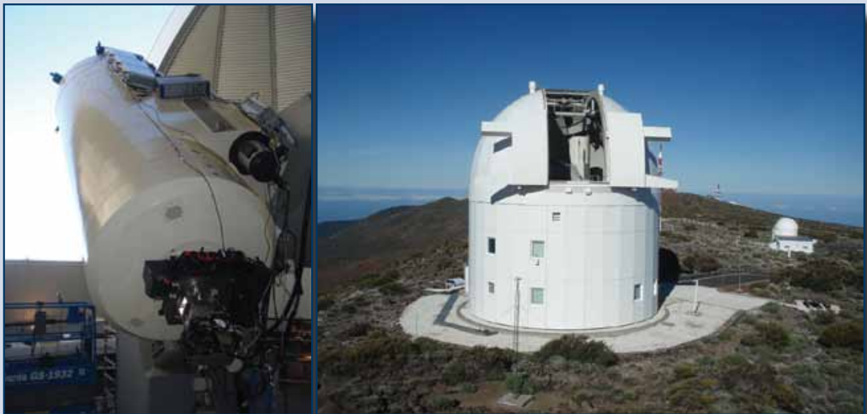
1-m OGS telescope with transmitter equipment (left) and OGS building with open dome (right).
