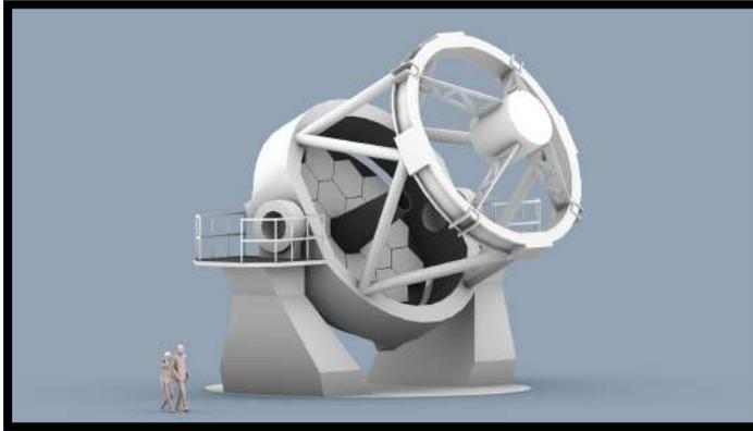
NRT will be a modern, 4-metre class facility located at the OOC and dedicated to time domain astrophysics with a focus on astrophysical transients, that aims to build on the success and experience gained with the Liverpool Telescope. This new robotic telescope with a 4-metre aperture will be a powerful tool for the study of supernovae, since the flexibility of robotic scheduling allows observing cadences to be optimised for each
